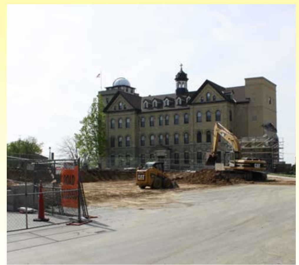
Construction crews begin digging for the foundation of St. Joseph Hall.
